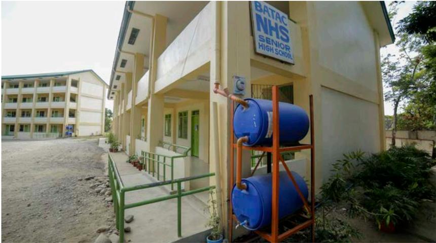
**Water-harvesting facility.** With their scarce water resource, the school actively harvested and saved rainwater. Along the school were canals that catch water and channel it down to the small water reservoir. The accumulated water is used in their vegetable plots, and a certain portion of the reservoir is utilized for tilapia production.
