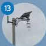
**Solar-Powered Street Lights.** They store electricity via lithium-ion batteries, which automatically switch on at night and can light up even in heavy overcast or rains for 3 days.
