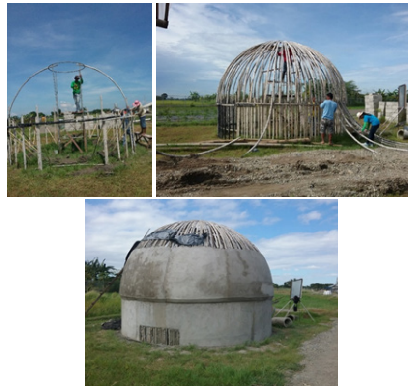
Figure 8. The farm structure constructed from a combination of straight and curved BCUs.
