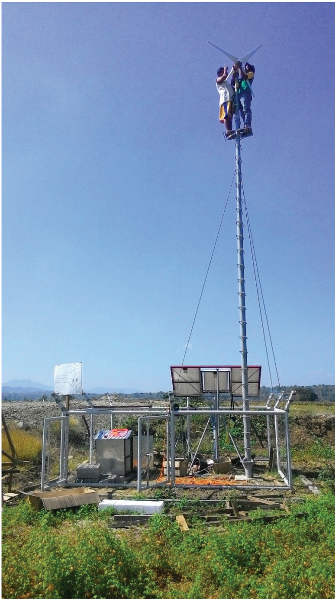
Figure 8. Installation of the 7.5 m high wind turbine tower.
