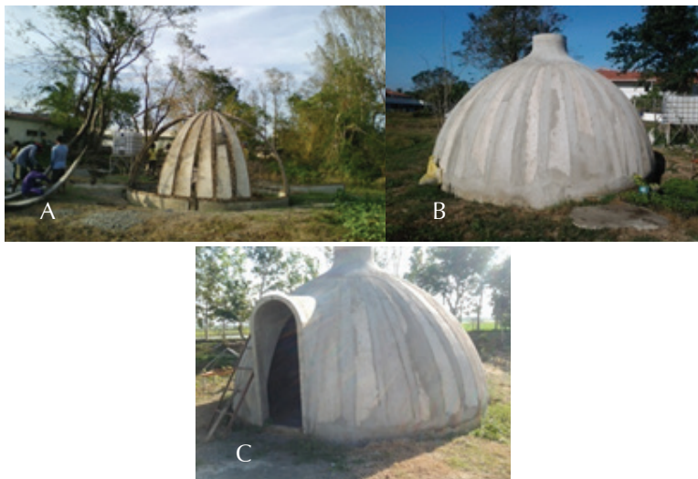
Figure 9. The multi-purpose farm structure during the start of assembling the BCUs (a) and when completed (b and c).
