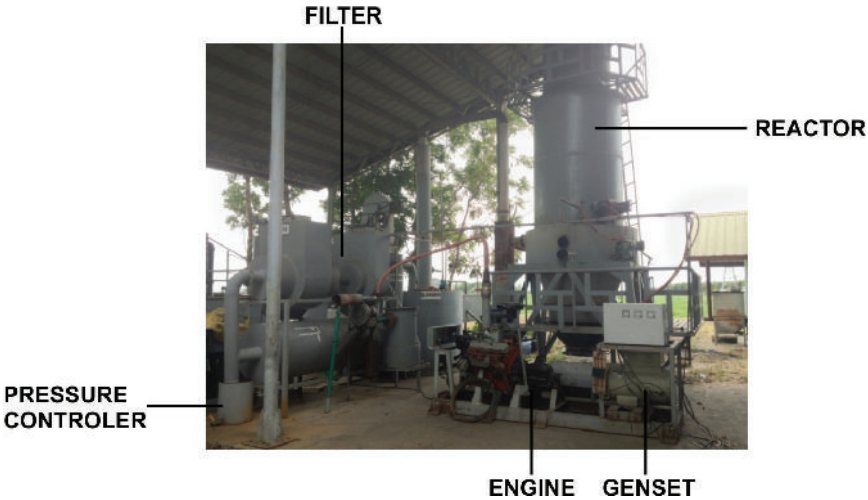
Figure 2. The 100kW rice husk gasification system
