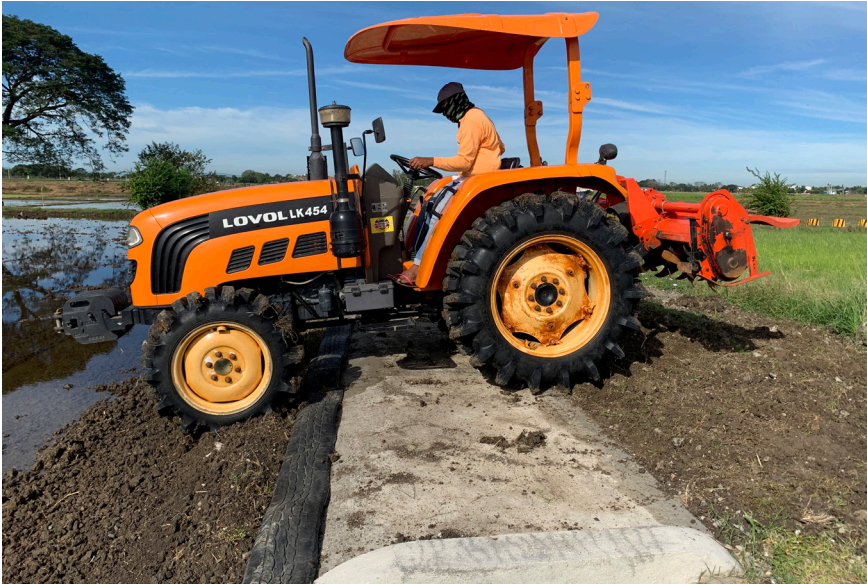
Figure 19. The concrete ramp with rubber lining at the REMD Farm.
