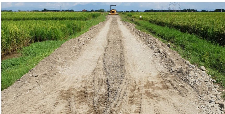
Figure 17. Graveling of access road at the REMD Farm.
